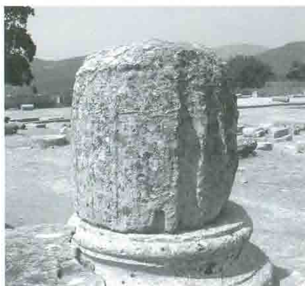
c. Block D54 with groove for clamp
