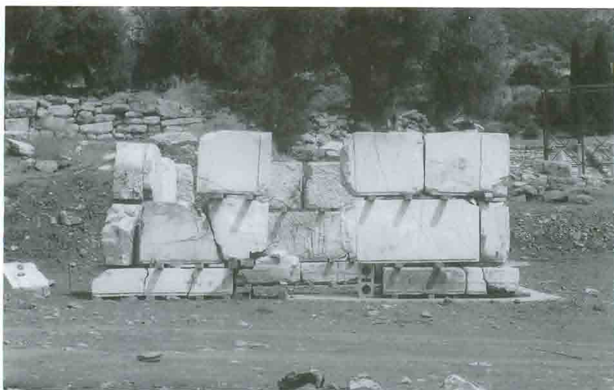
Pl. 49 K3, Lower part of the wall
