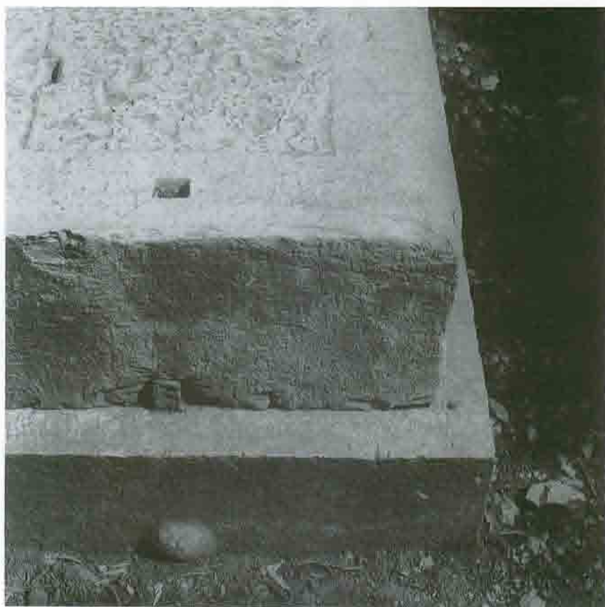
Pl. 30 K3, Dowel and dowel hole on the southwest corner
