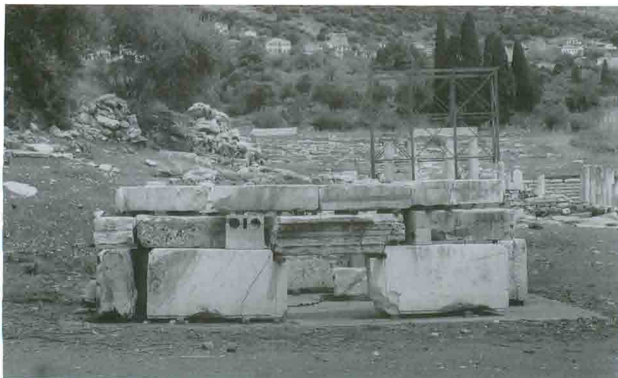
Pl. 48 K3, Upper part of the wall
