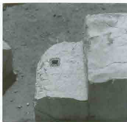
Pl. 32 K3, Wall block with a dowel hole fixed with lead (XI.73)
