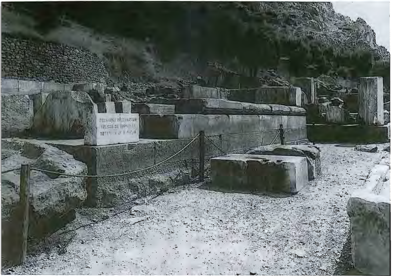
Pl.1-5 Front view from the southwest
