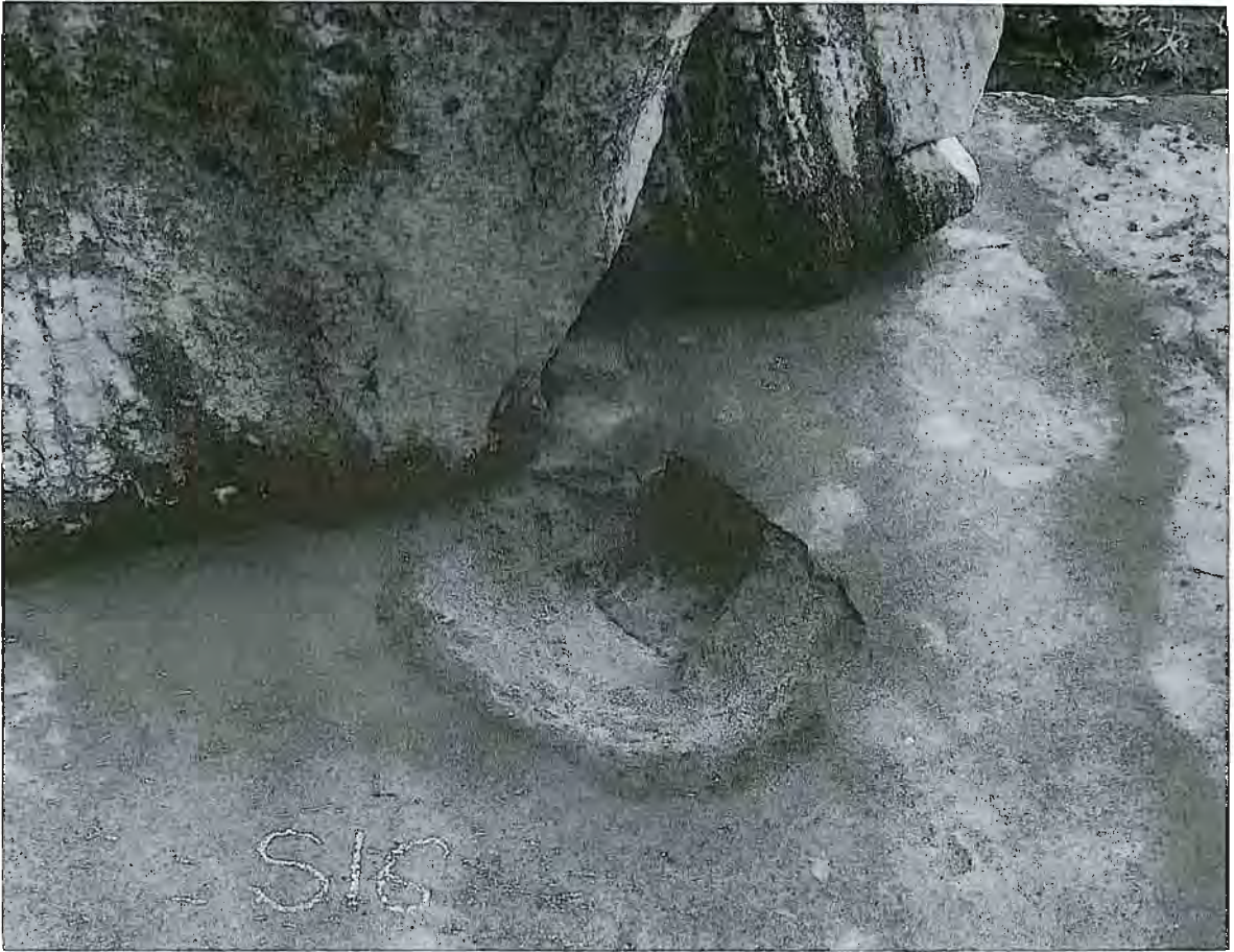
Pl.3-32 Dowel hole of a column (S16)
