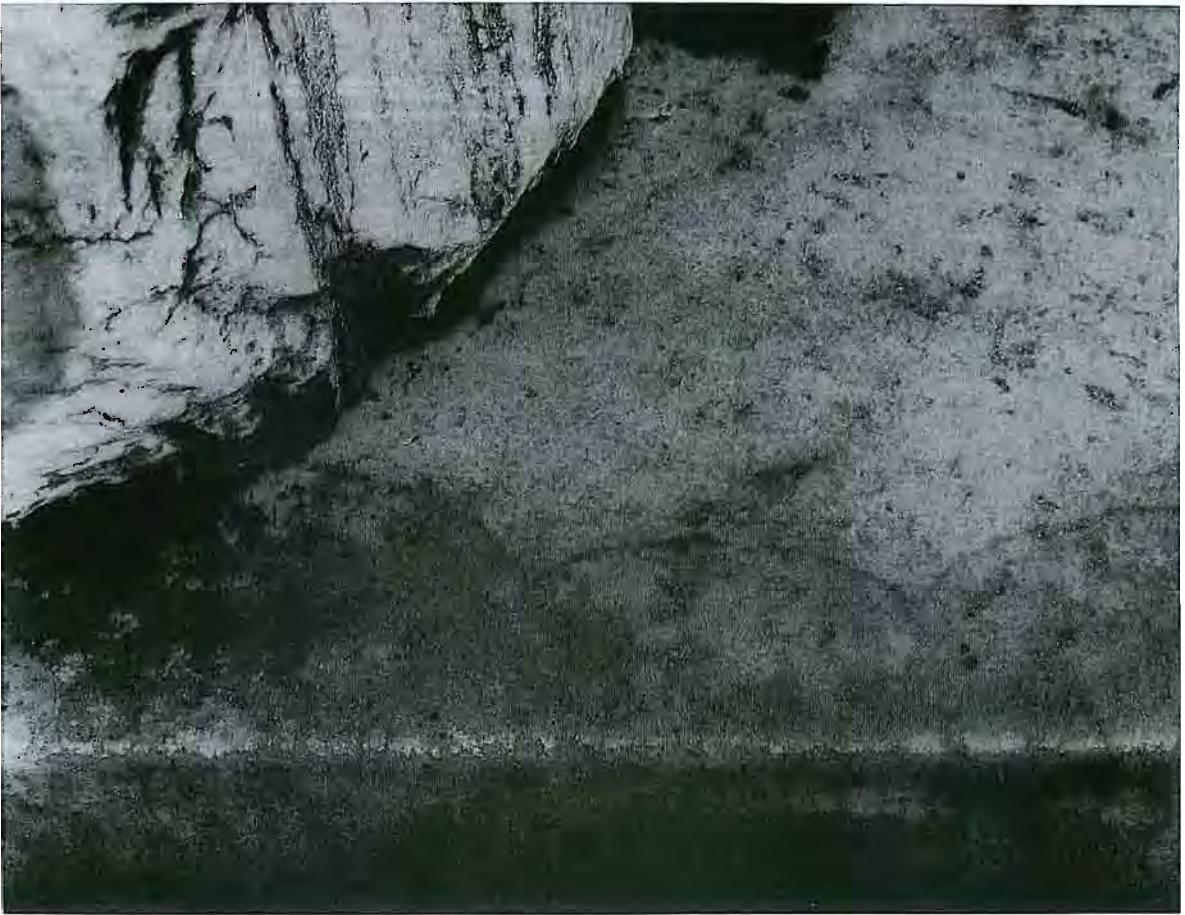
Pl.3-30 Setting line and fluting line of a column on the stylobate (S34)
