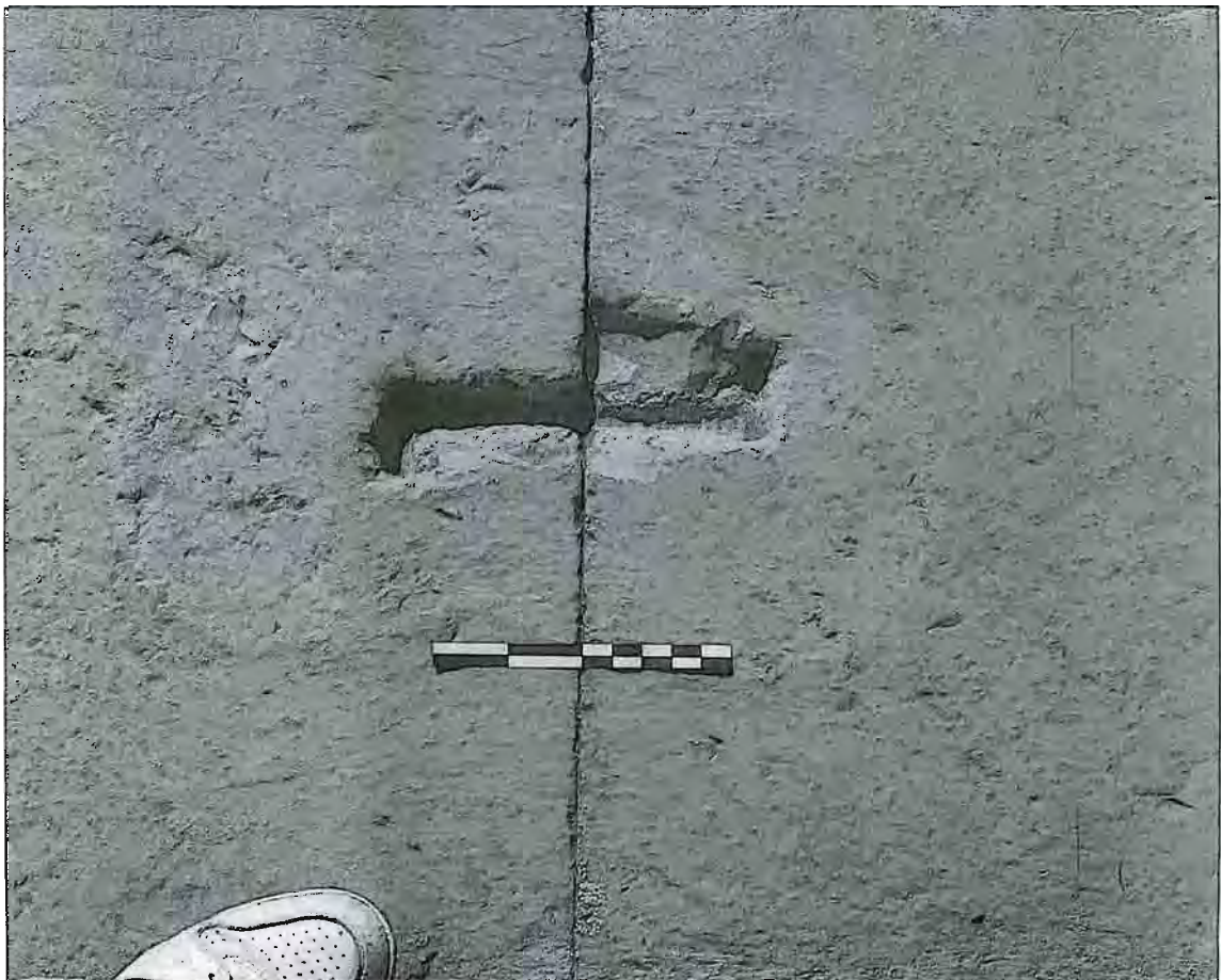
Pl.2-33 Trace of double- \Gamma clamp on the west euthyteria
