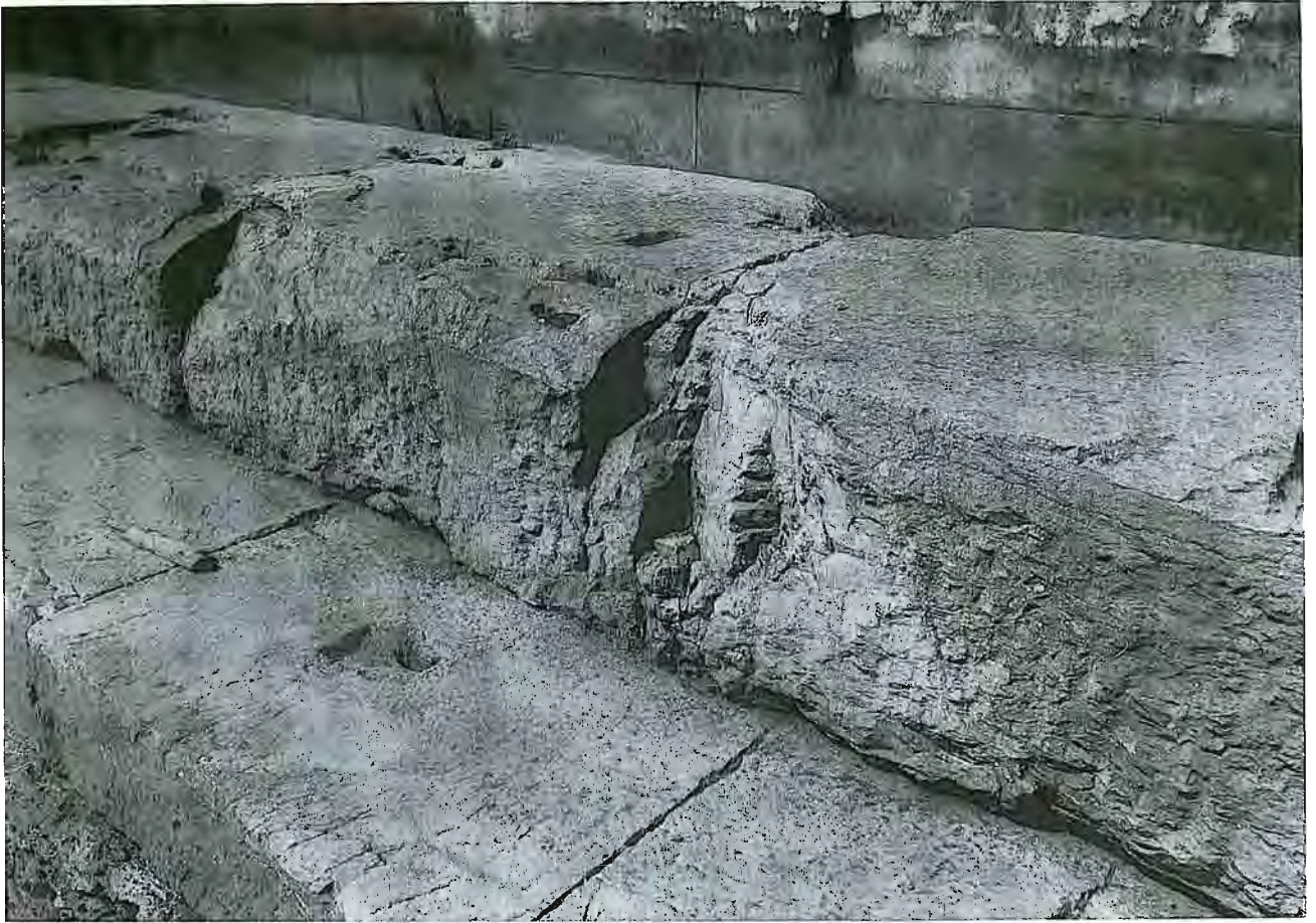
Pl.1-59 Breaking off of limestone blocks of the bench of the naos
