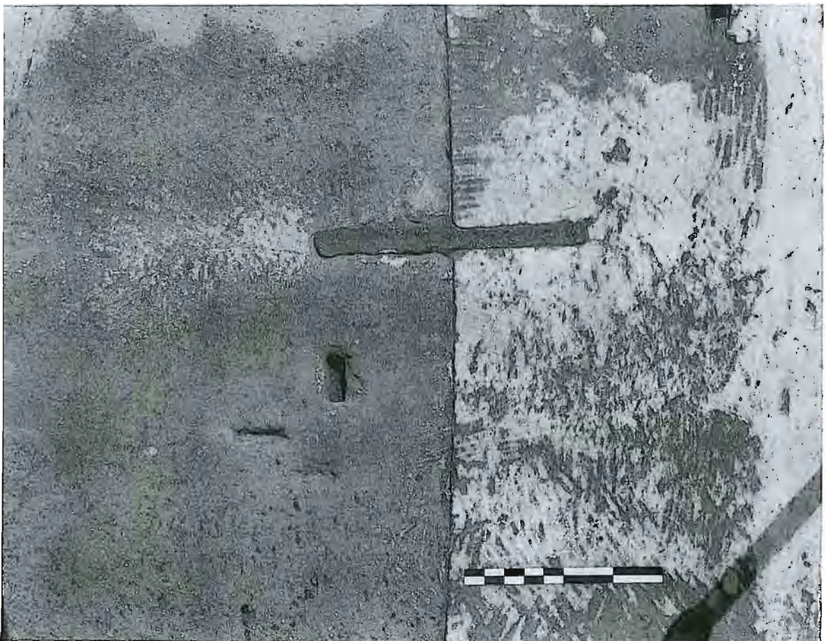
Pl.3-37 \Pi -shaped clamp, dowel hole and pry holes
