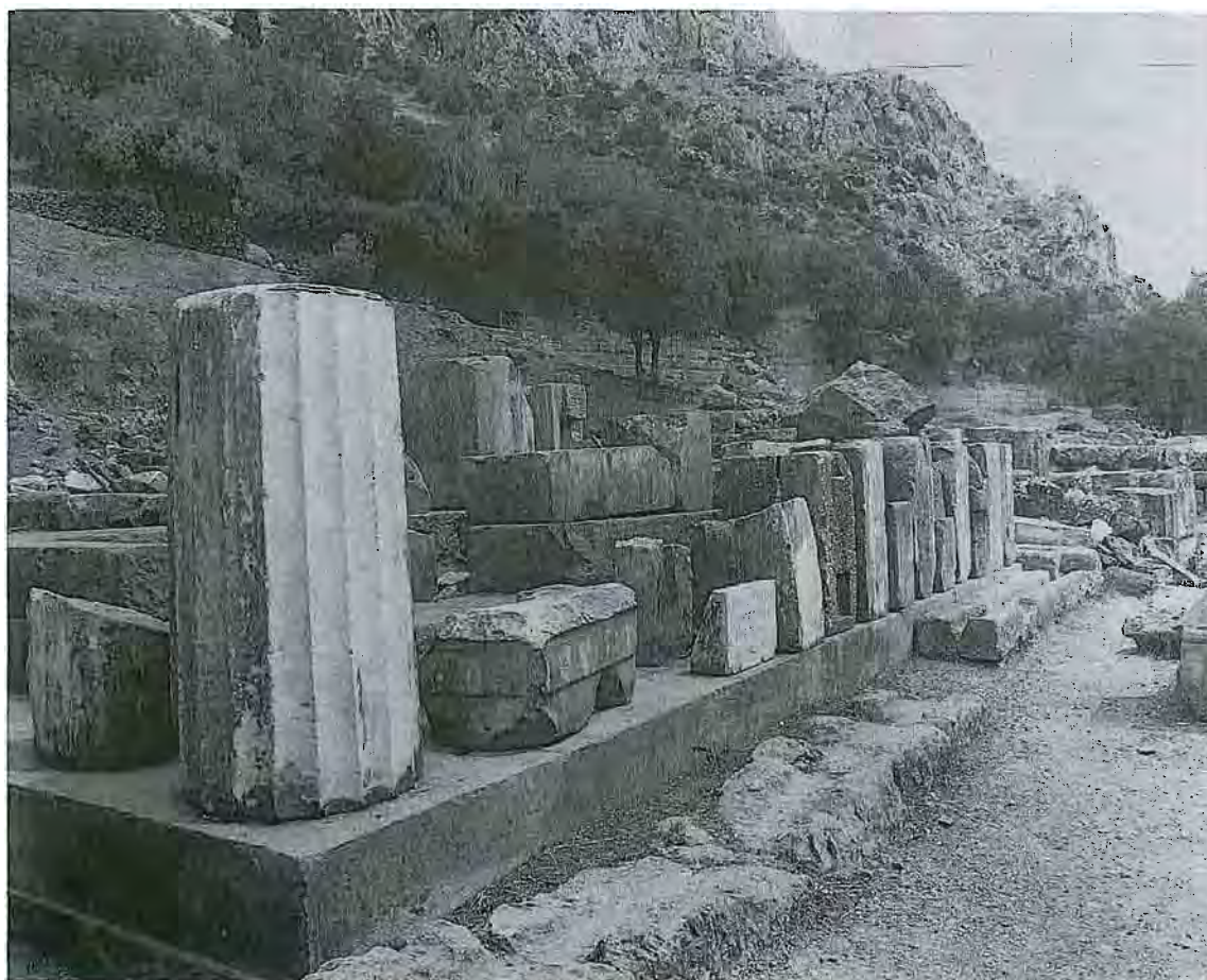
Pl.2-4 Front view from the southwest
