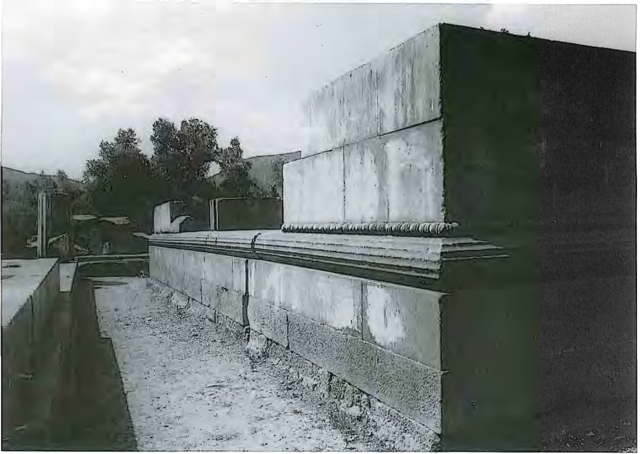
Pl.1-11 East side view from the north
