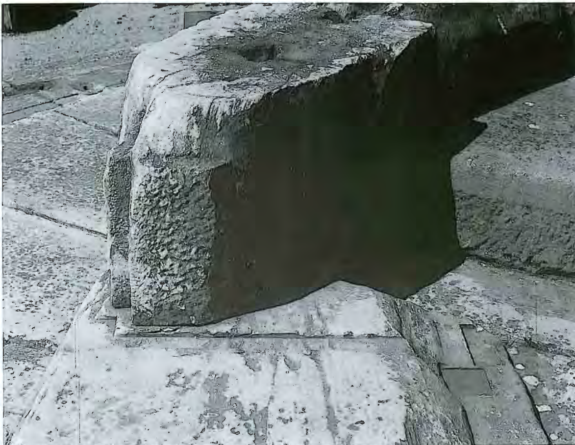
Pl.3-16 Detail of threshold
