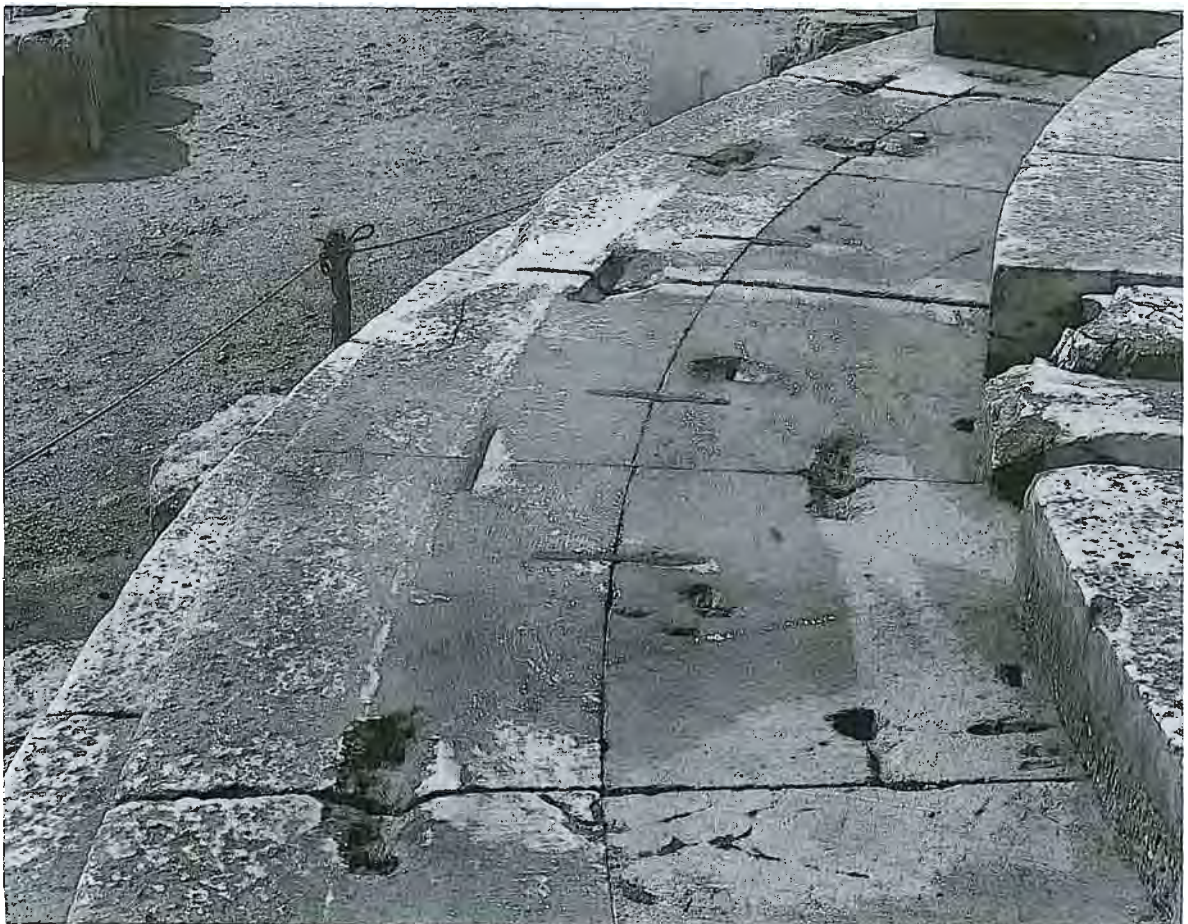
Pl.3-33 Traces of clamps and pry holes
