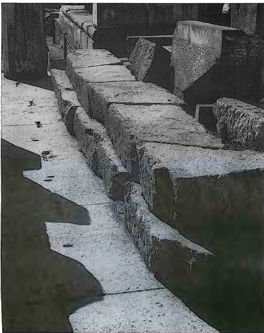
Pl.2-15 Front foundation and euthynteria
