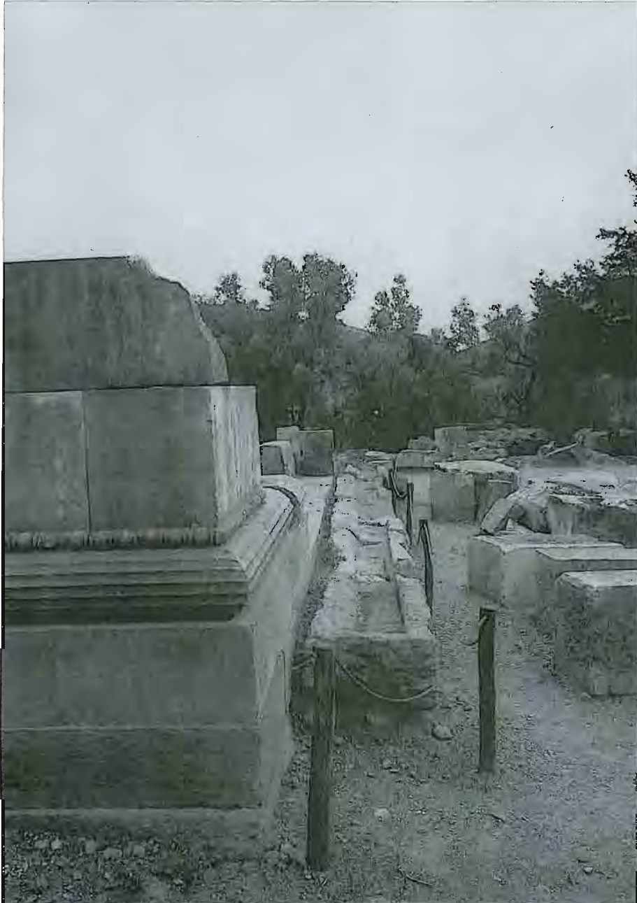
Pl.1-18 Northwest corner and the east side
