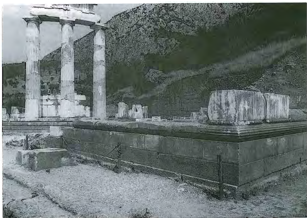
Pl.1-4 Front view from the southeast
