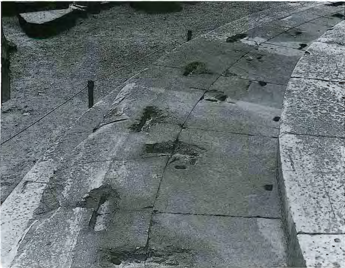
Pl.3-34 Traces of clamps and pry holes
