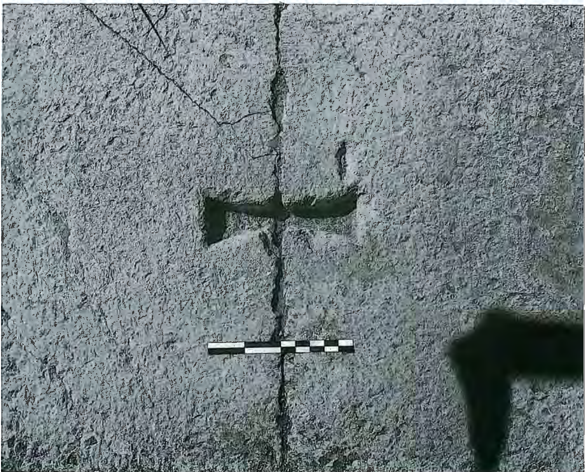
Pl.2-35 Trace of dove-tail clamp on the cross wall foundation
