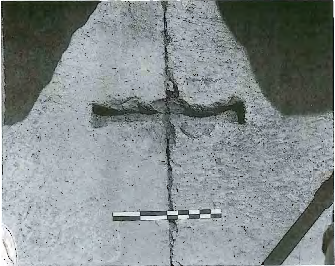
Pl.2-32 Trace of dove-tail clamp on the front euthyteria
