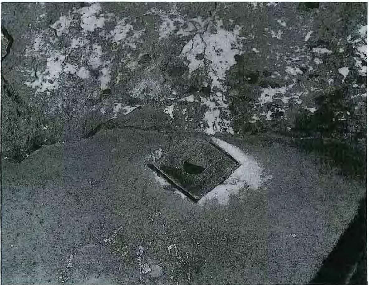
Pl.3-31 Dowel of a column on the stylobate (S20)
