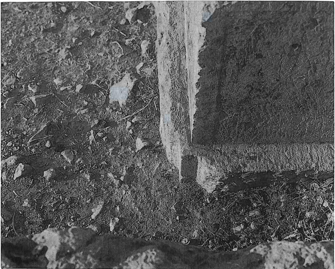
Pl.2-18 Detail of west corner
