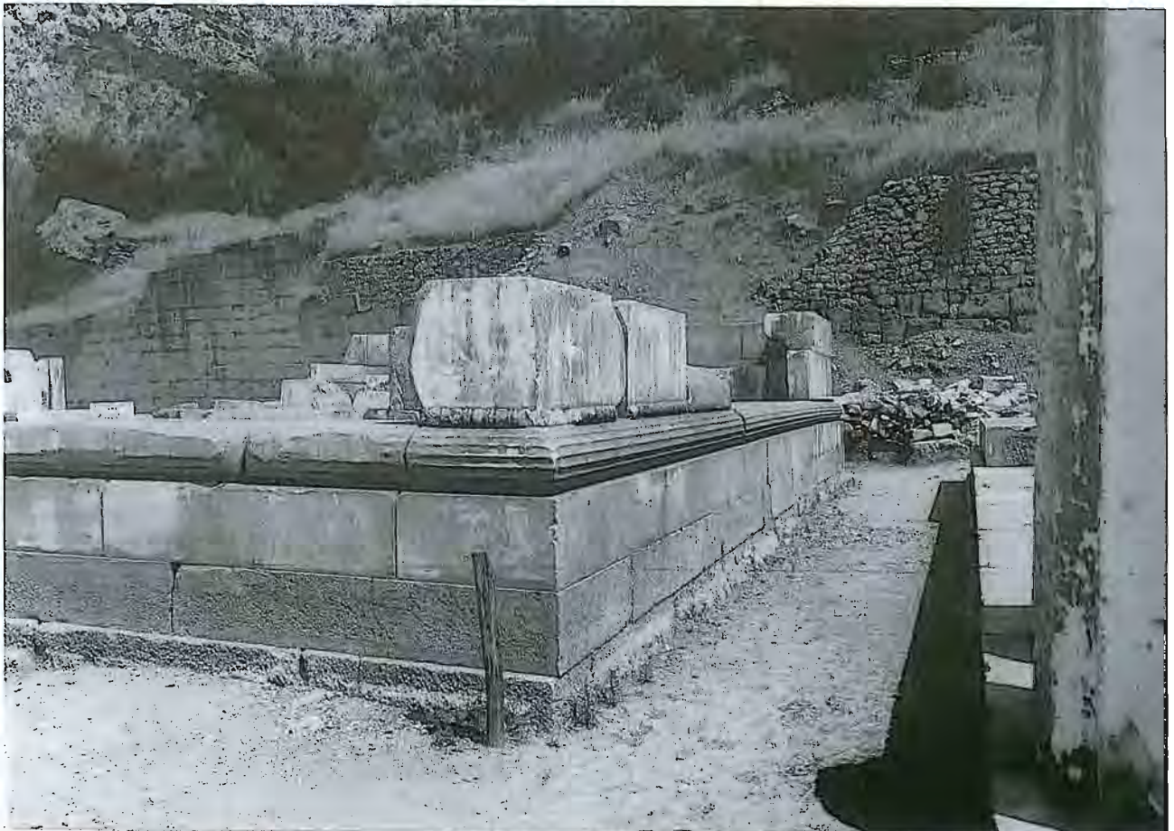
Pl.1-10 East side view from the south
