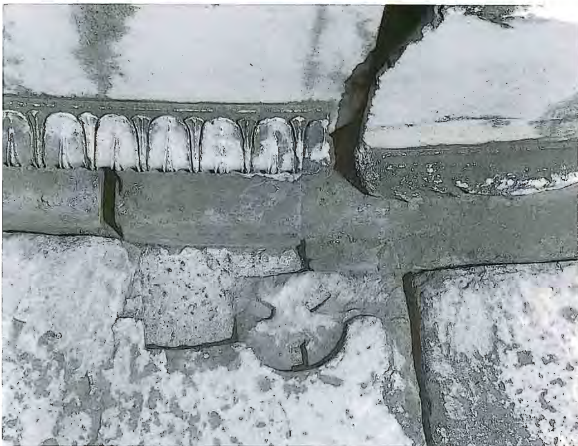
Pl.3-19 Detail of doorway
