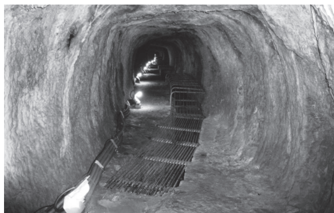
Fig. 3 View of the tunnel, about 65 m from south entrance (near S105)
