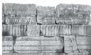
Fig. 13 Jerash, the entablature and geison of the west facade of the west Propylaeum of Artemision
