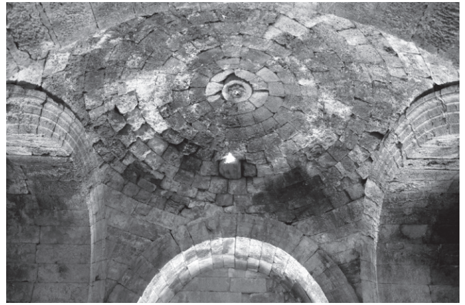
Fig. 9 Amman, domical vault with pendentives of Nuweijis, looking from the northwest to the southeast
